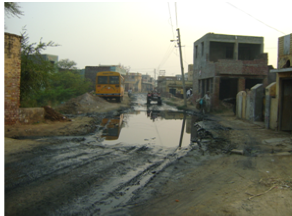
Stagnation of waste water and rain water due to
